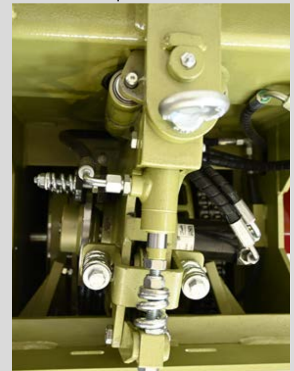
■ Hydraulic cable ejector with cable dispenser
